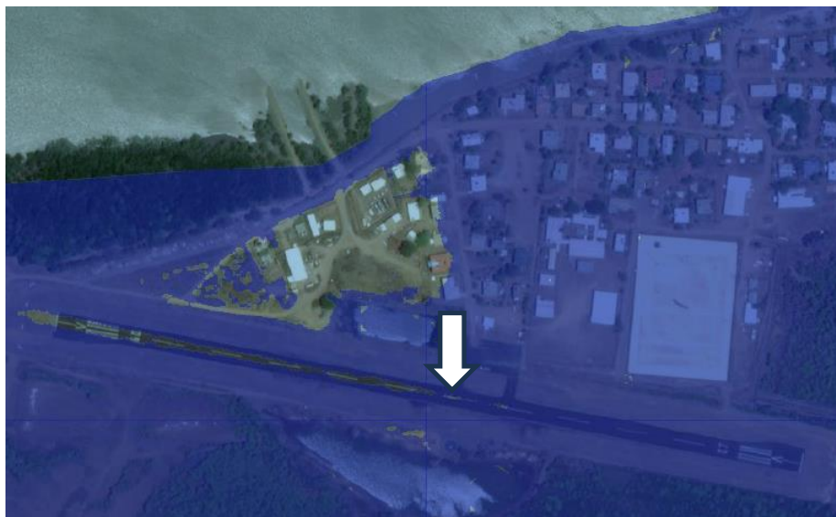
Figure B – Extract of BR Fig 12 (p25) with location arrow and shaded 3.73 m AHD level just showing the exposed airstrip centreline in the proximity of Figure A.
